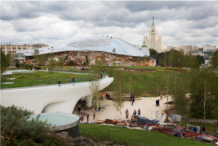
Zaryadye Park. Under construction, summer 2017.
